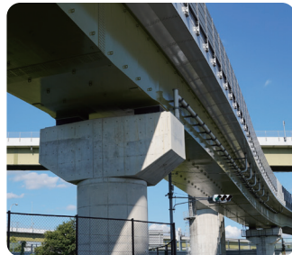
Highway Side Walls
