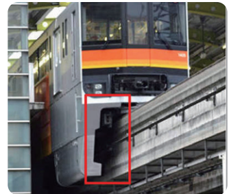
Guide Rails of Monorail Tracks
