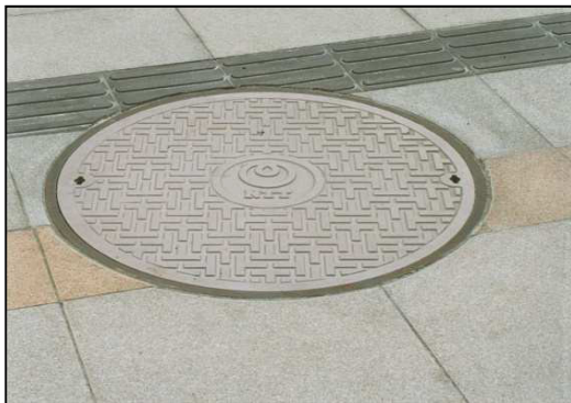
Anti skid manhole covers
