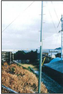
Steel poles (echo)
