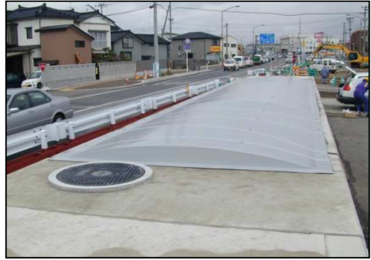
Bridge Utility Fixtures (additional fixtures)
