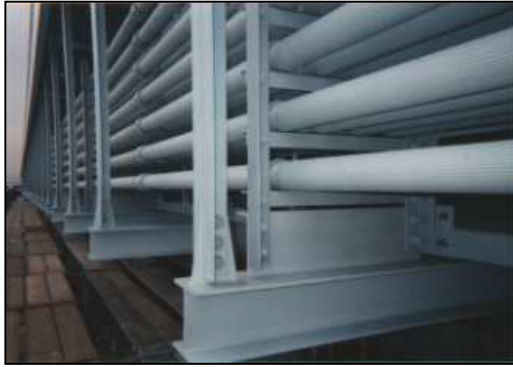
Bridge Utility Fixtures (Main units)
